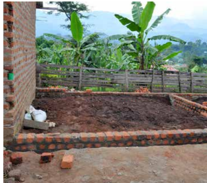
Above: Foundations for new classroom at Kirindi School
