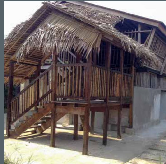
Above left: Tinangol kindergarten. Concrete support struts have now replaced wooden poles
