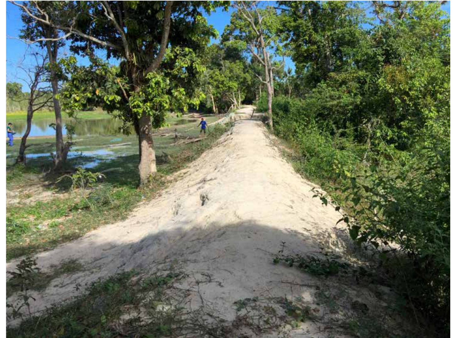
Above: Wall of Ta Lek dam, reinforced by our volunteers
