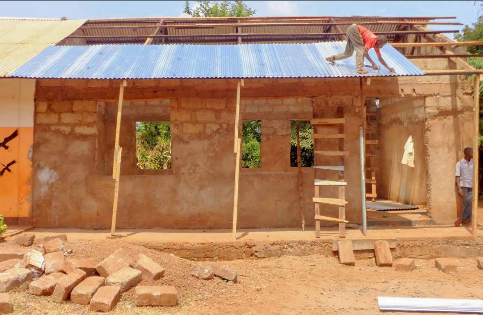
Above: Classroom construction at Father Neville School
