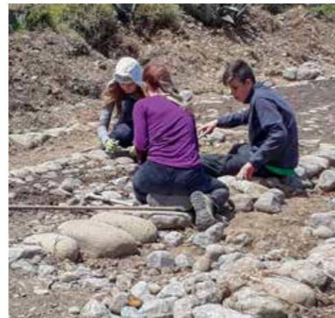
Above: Paving the road to Kuri Kucho
