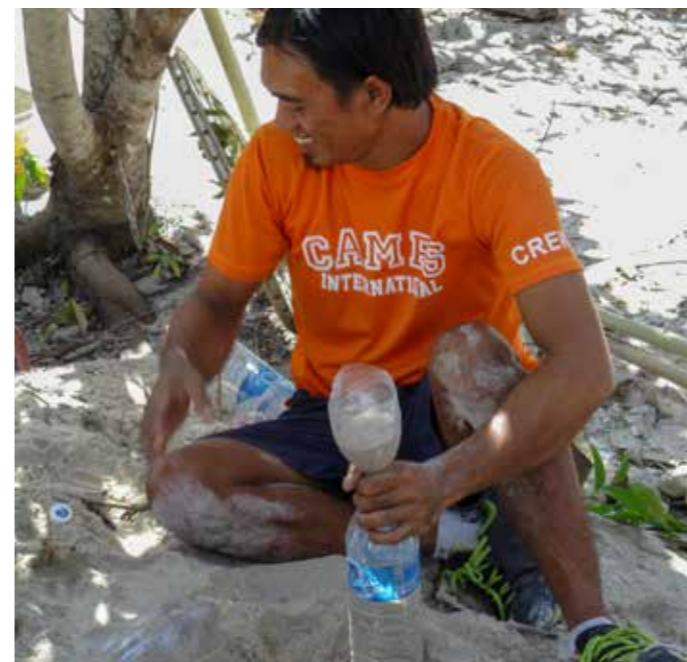
Above left: Filling discarded plastic bottles with sand to be used in constructing the recycling hut.
