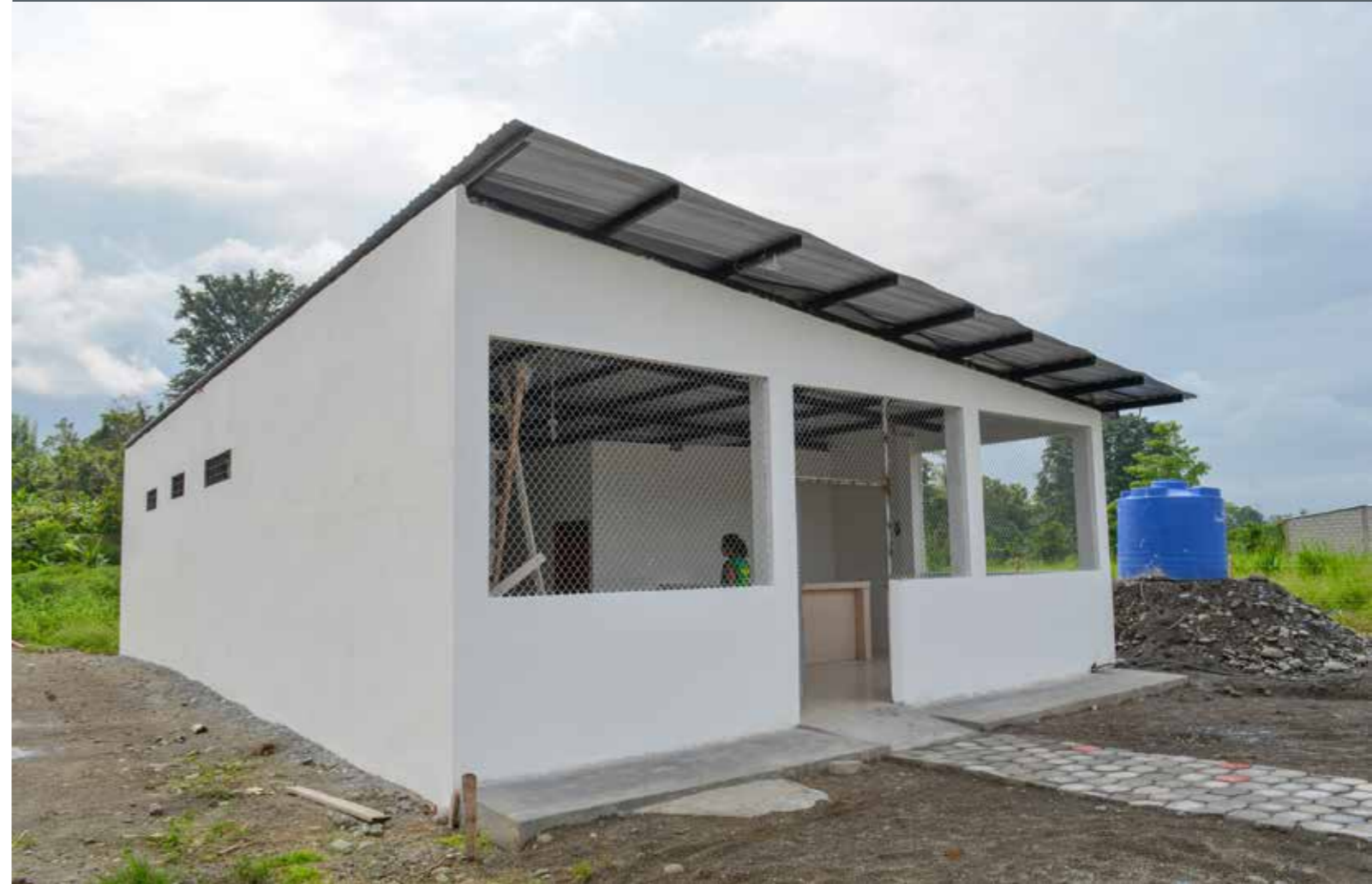
Above: New Medical Centre (now complete)
