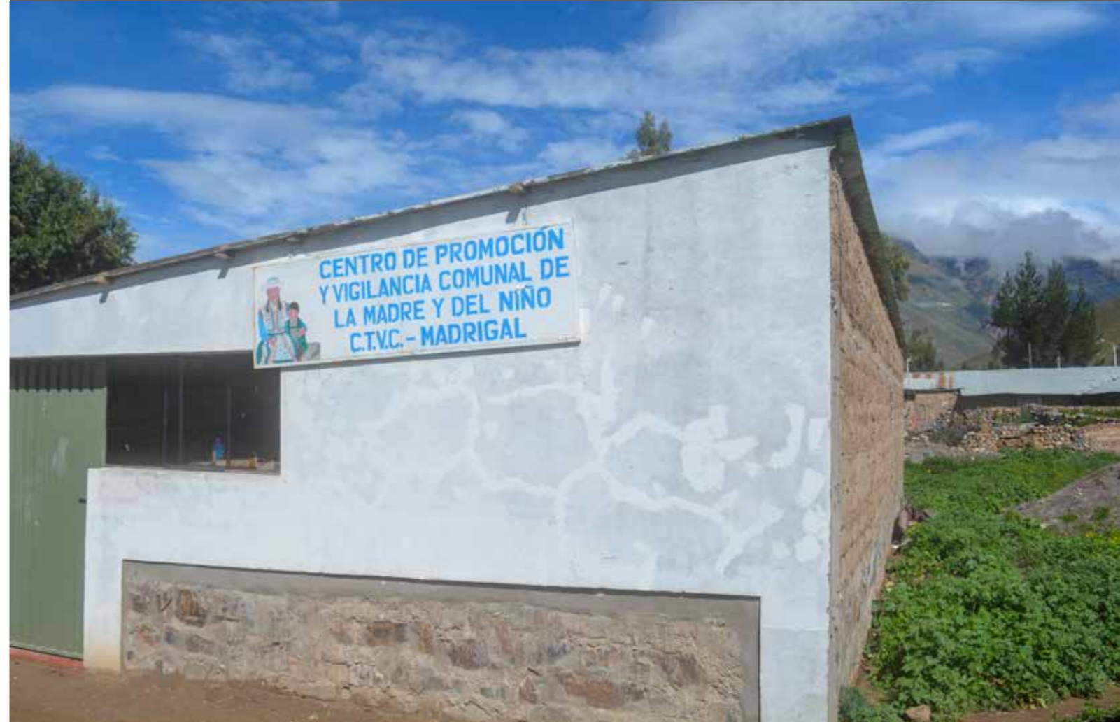
Above: New kitchen and prenatal centre. The land shown to the right of the building is the proposed site for the community elders meeting room (PC-COL-004)
