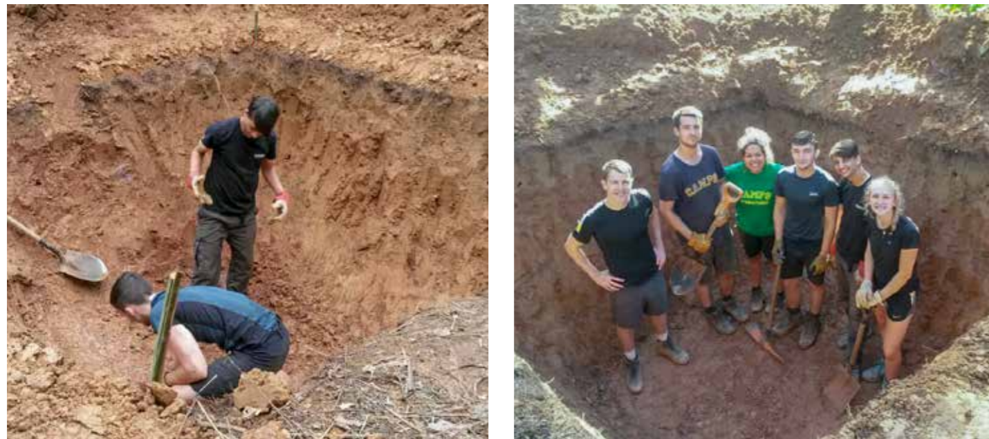
Above: Excavating the new community reservoir at Chilly Urku
