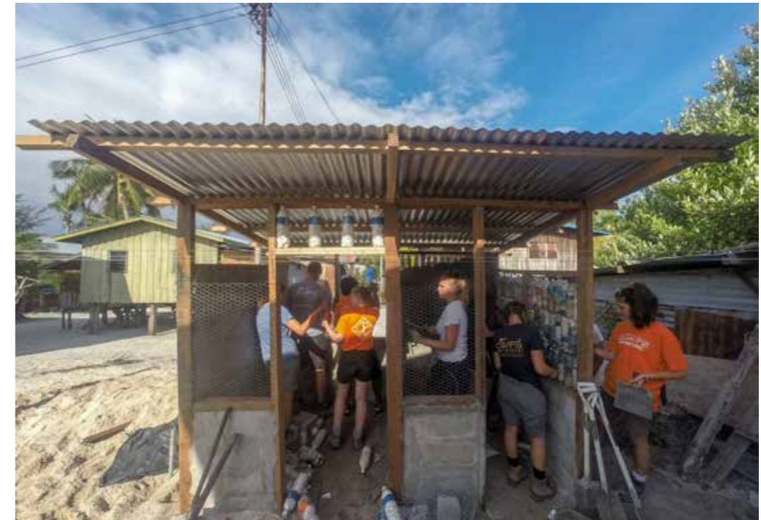
Above: New toilets at Mantanani
