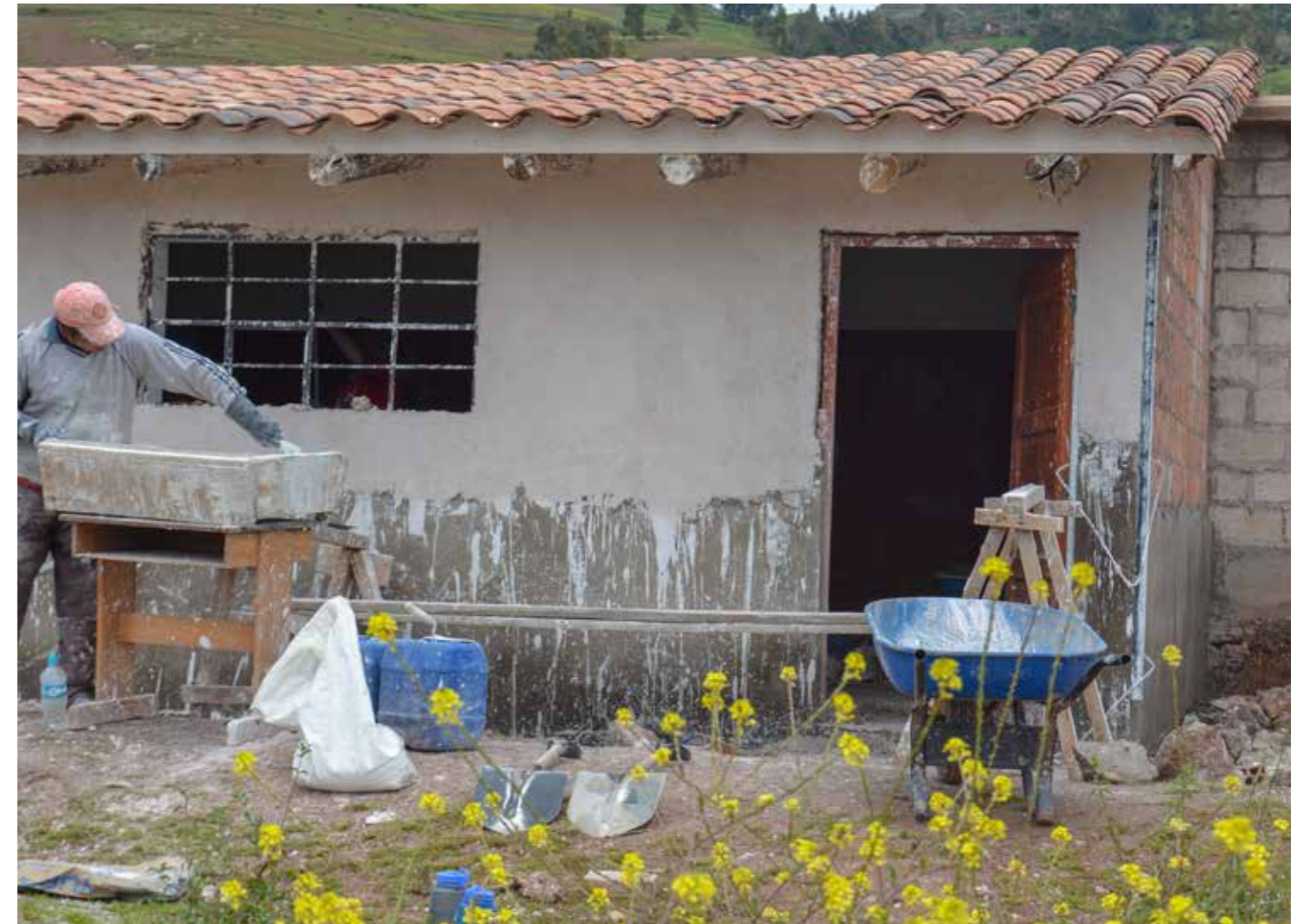
Above: New kindergarten under construction at Anqoto
